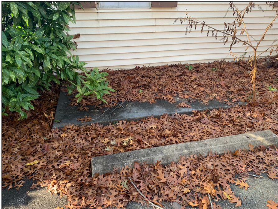
14 - Concrete pad located along the eastern side of 454 N Madison Road
